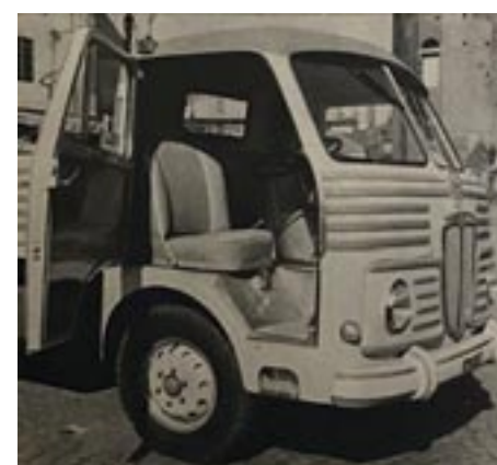
Final series, the 190 Z50, built until 1961 with Viberti's updated and reinforced cab, 'cat's whiskers' front, and repositioned turn indicators, available only in one length/width configuration.
