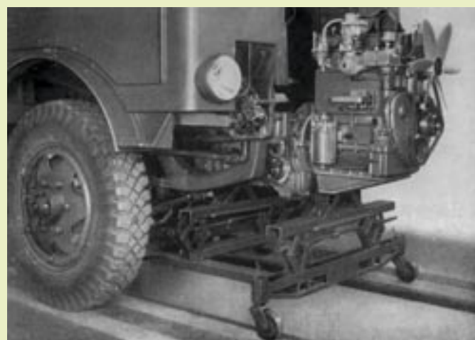
The engine (shown above without cover) could be dropped and then pulled forward for ease of servicing and maintenance, an important factor for the Z20 (CL51) military model.
